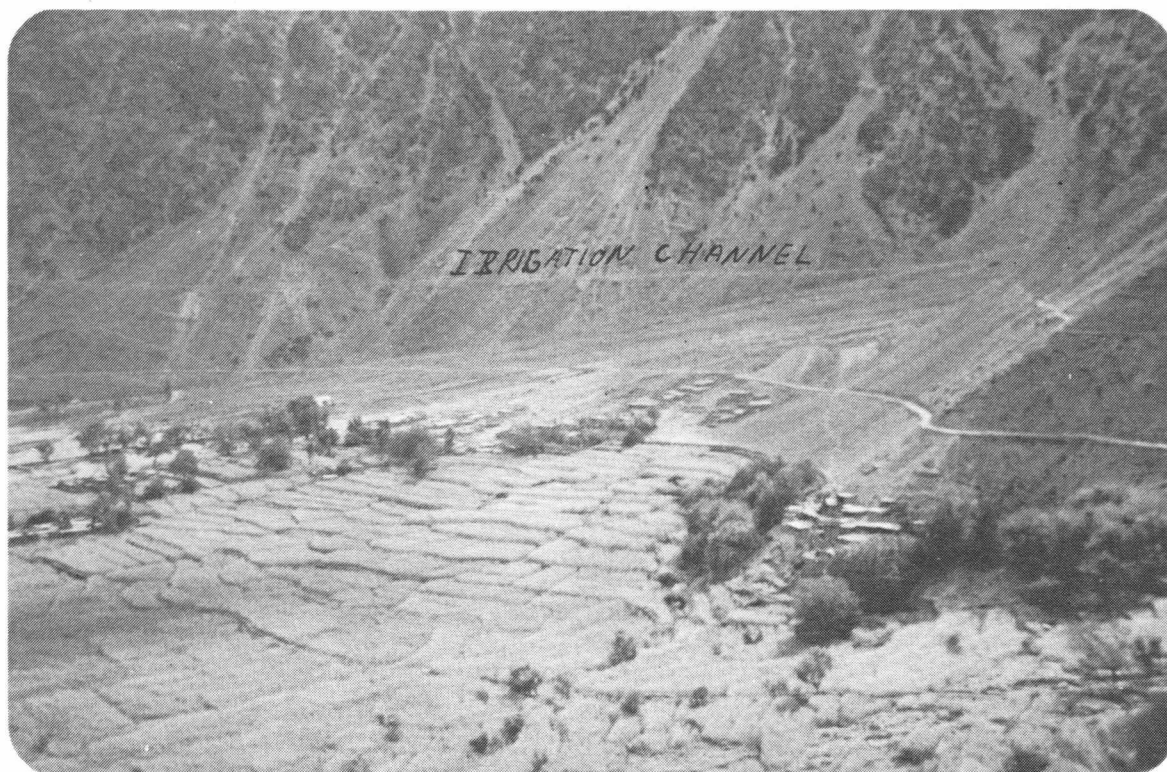
The settlement of Luruk, Tangir. An irrigation channel is constructed in the hillside. The main channel from the river, however, cannot cater for the necessary amount of water for the whole area.
