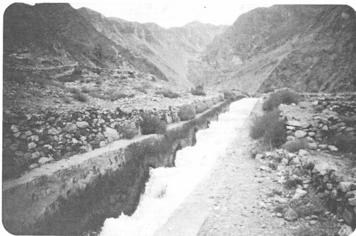
Cascade in feeder channel for Nomal hydel power plant.
