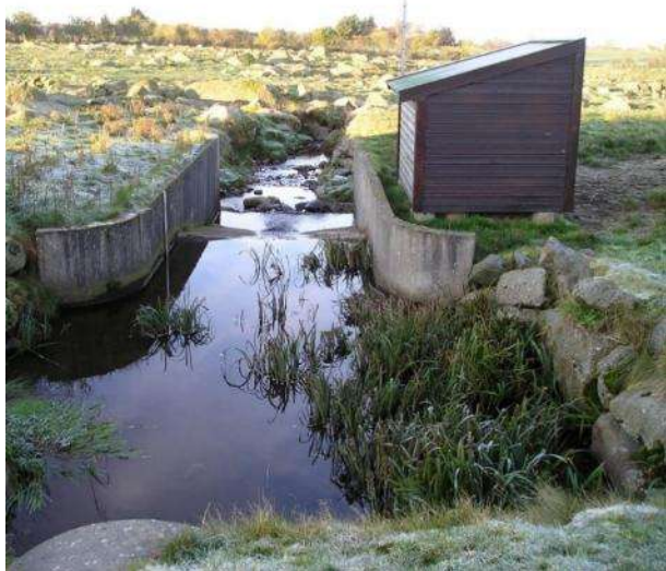
Figur 8-51: Begroing i oppstrøms basseng (Foto: NVE)
