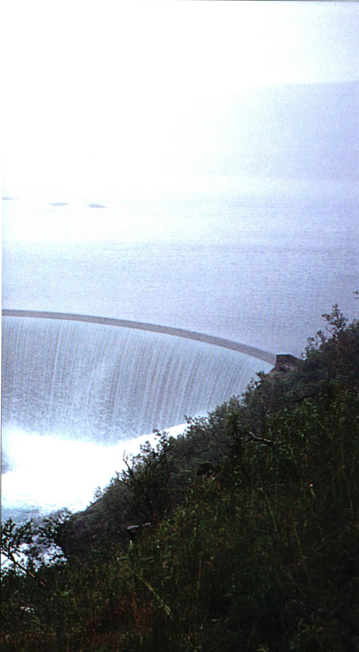
THE SPILLWAY OF A RESERVOIR DAM (HOLMVASSDAMMEN) IN NORTHERN NORWAY. PHOTO: ARNE H. ERLANDSEN.
