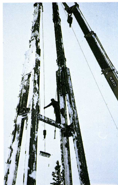
Limtremast under montering.
