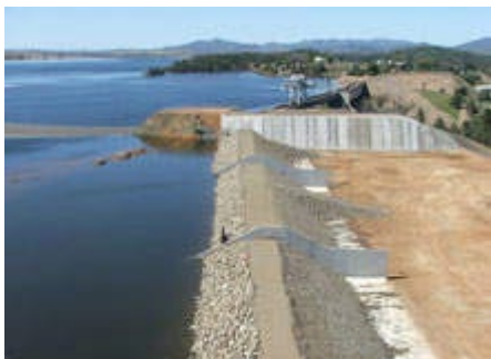
Figur B 22 Eroderbart flomløp etablert ved Keepit dam, New South Wales, Australia. (Figur fra: https://www.power-technology.com/projects/keepit-dam-safety-upgrades-new-south-wales/?cf-view ).
