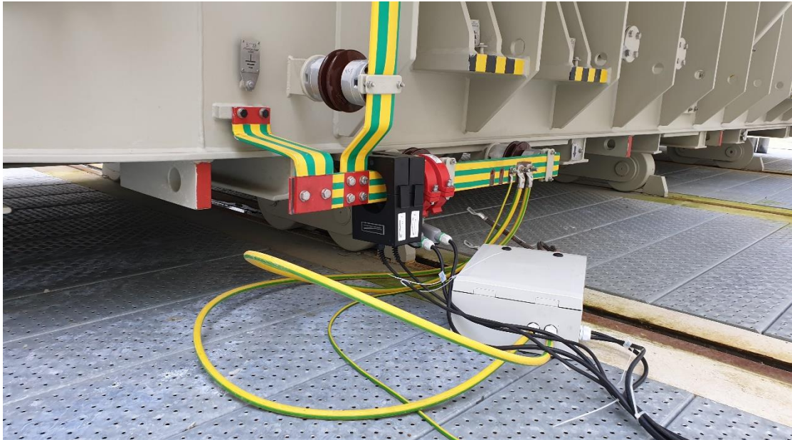
Figure 3-1: Four GIC-sensors (2 black and 2 red) on transformer neutral. Regular hall effect sensor in grey box, see Figure 3-2.
