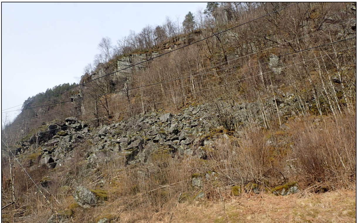
Figur 8 Steinsprangur aust for steinskredura.
