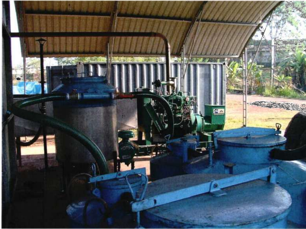
Wood Gasifier - Internal Combustion Engine Driven Generator (Sapugaskanda)
