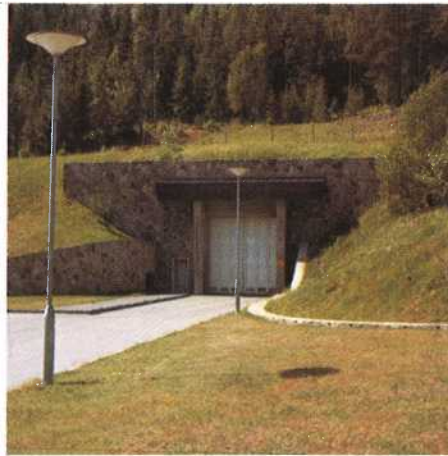
Entrance to a power station.
