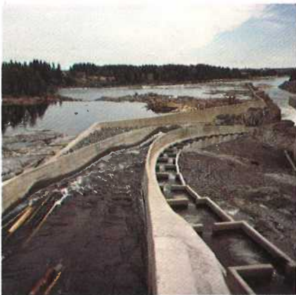
Timber slide and fish ladder.
