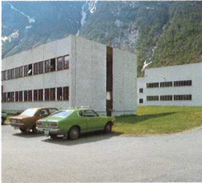
Administration building and workshop at a power construction site.
