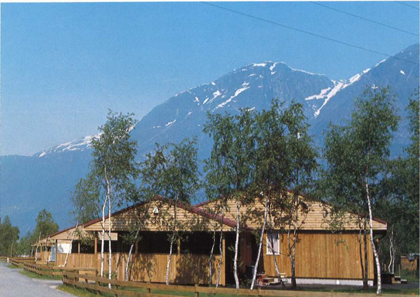
Housing area at a power construction site.
