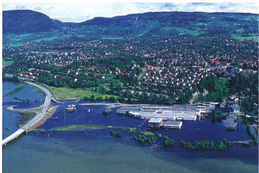
New shopping centre, flooded during the 1995 flood. The flood resulted in a recognition of the need for improved land use planning in flood prone areas and improved emergency preparedness. Photo: Fotonor
