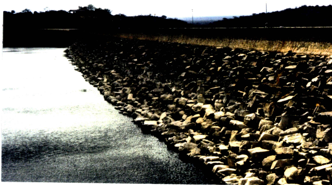
Day 5 - Upstream rock protection at Nyumba ya Mungu Dam
