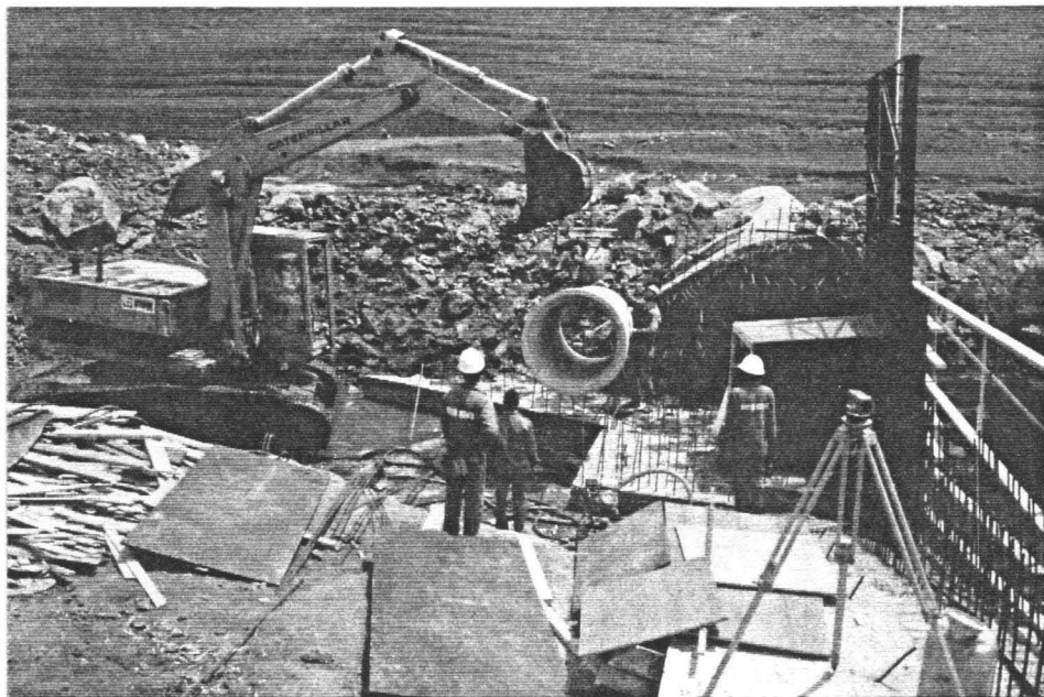
Erection of first pipe section at intake, December 1986
