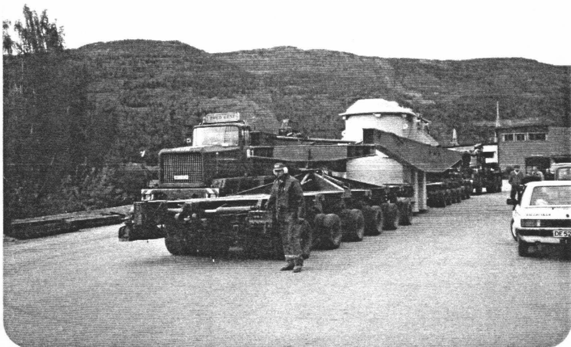
Transformatortransport 1989. 110 MVA trefase transformator.
