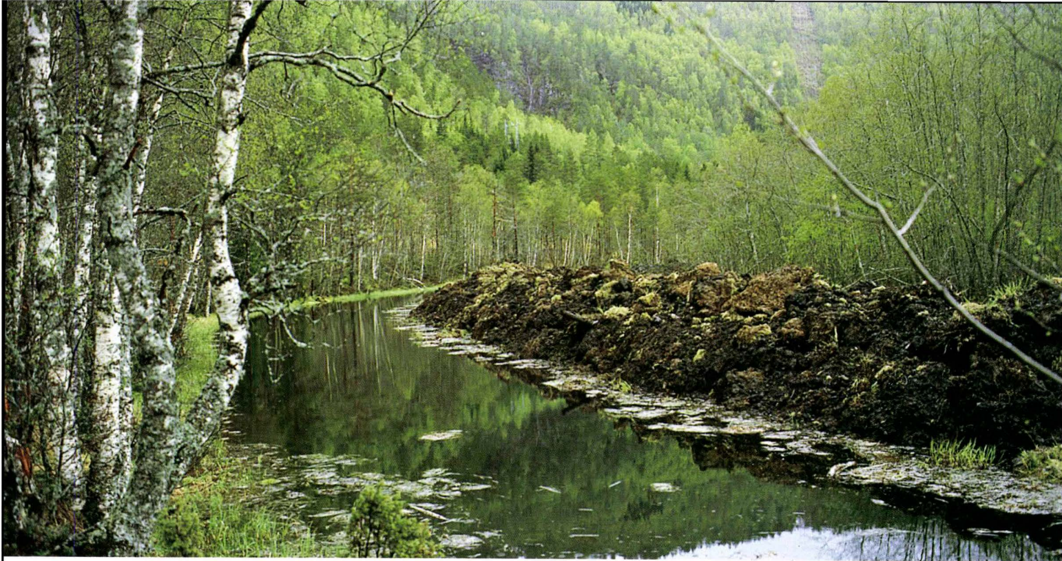
A meander in the Soya River soon after it was excavated in May 1987. Attempts were made to improve conditions for birds and fish by deepening the old meander and building man-made islands (photo: Jon Arne Eie).
