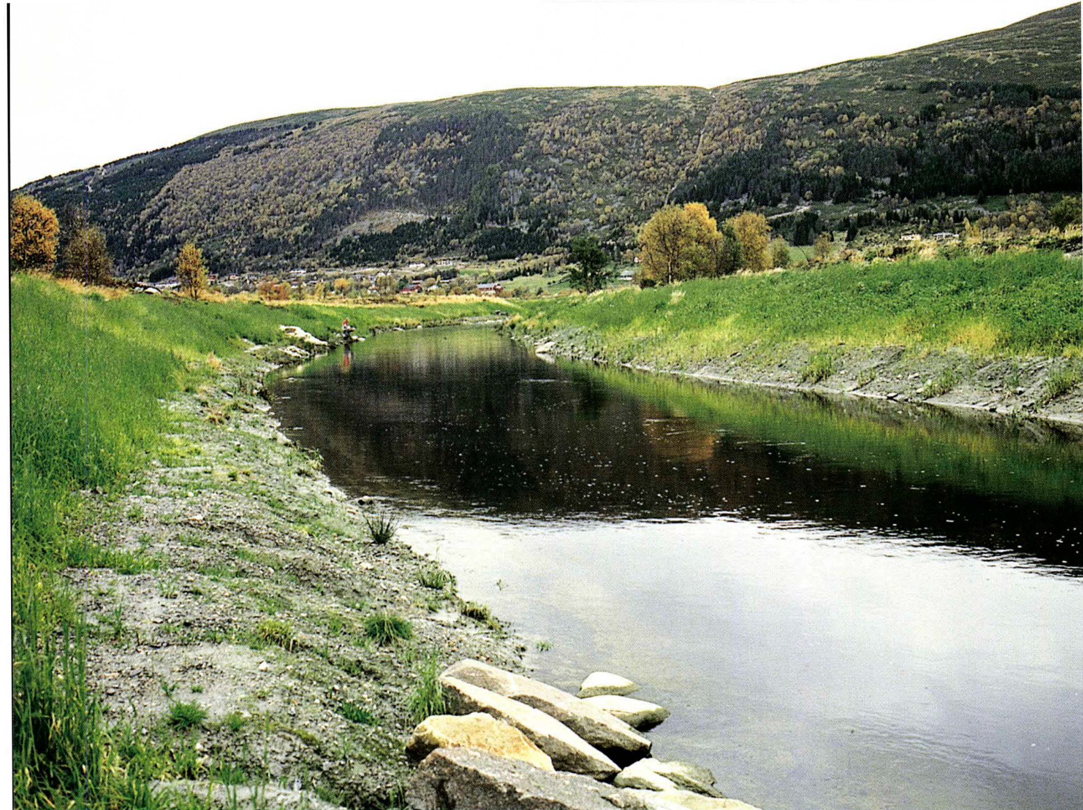
The banks of the channelized stretch are terraced to make the river more accessible for fishing both at low and high water levels. On the left, a fishing path for use when the water level is low. When the water level is high fishermen stand up on the earthworks. The riverbanks have been sown. The river, Hareidselva, October 1985 (photo: Jon Arne Eie).
