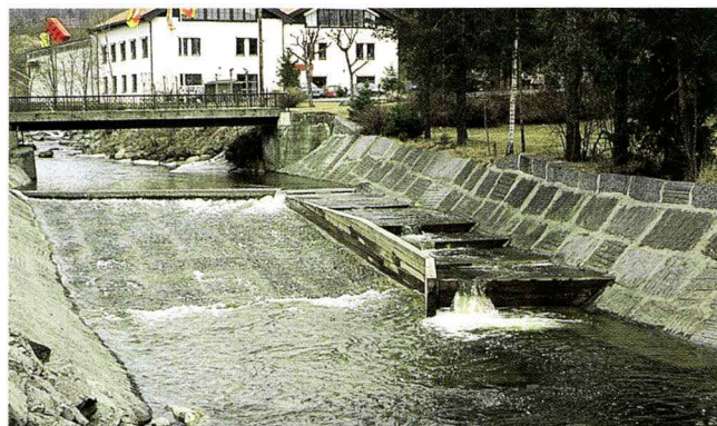
Concrete weir with a fish ladder in the river, Sandvikselva, April 1996 (photo: Jan Henning L'Abée -Lund).
