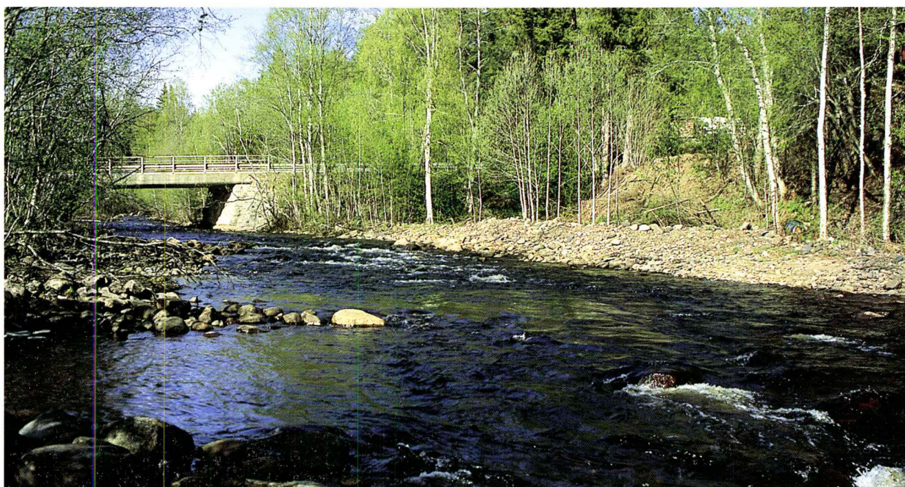
Biotope adjustment measures in Letjenna in May 1993. In the middle of the picture, there is a pool that has been excavated and current concentrators above and below it create riffles (photo: Jon Arne Eie).
