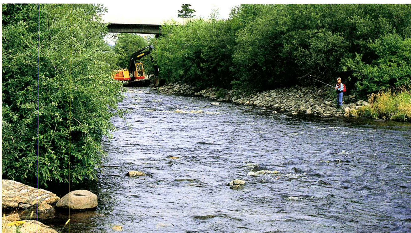
Biotope adjustment measures in the river, Brumunda, August 1989. The substrate was made more variable (photo: Jon Arne Eie).
