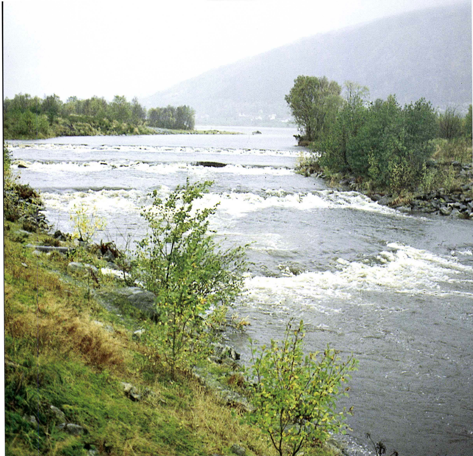
Weirs in the river, Hareidselva, below the lake, Grimstadvatn. The weirs were built to prevent lowering of the level of the protected Grimstadvatn and to safeguard the abundant bird life when the river was going to be channelized for agricultural purposes (photo: Jon Arne Eie).
