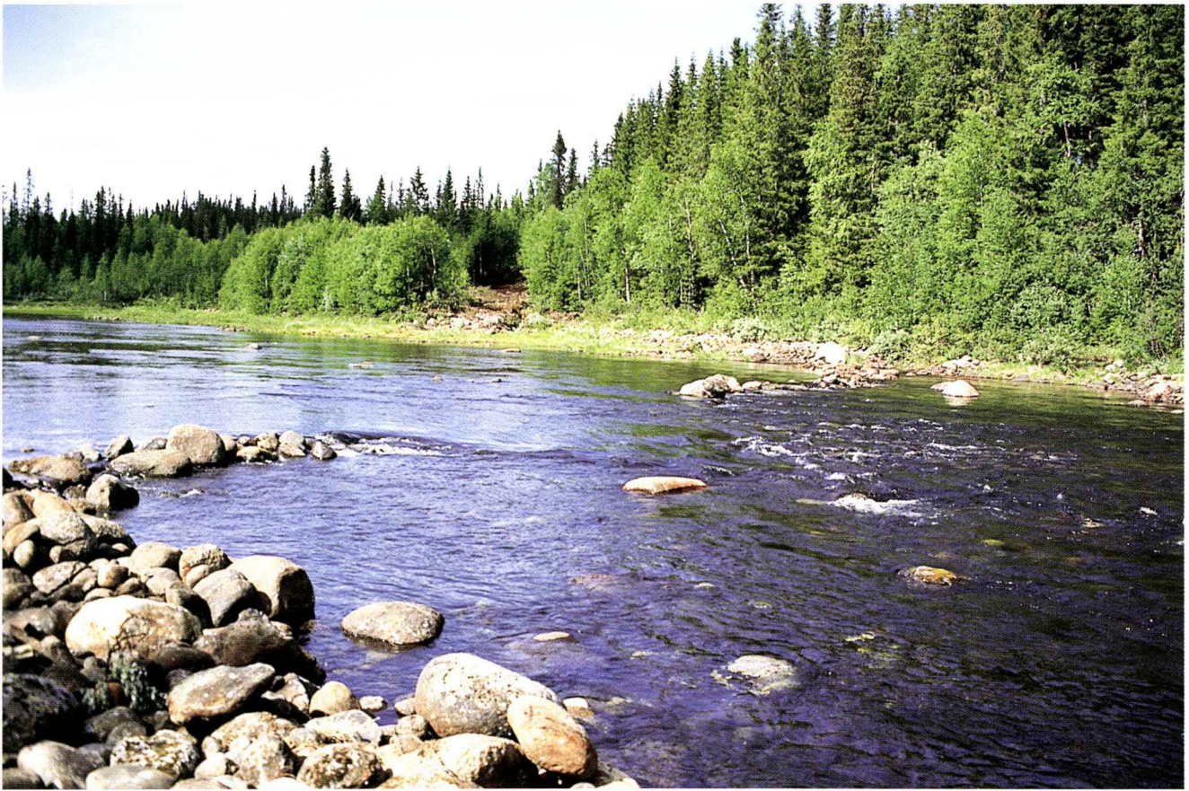
Biotope measures in a river in river, Umeälven, Sweden, with reduced flow. Pools have been made and rocks deployed to create riffles and cover for fish. June 1992 (Photo: Jon Arne Eie).
